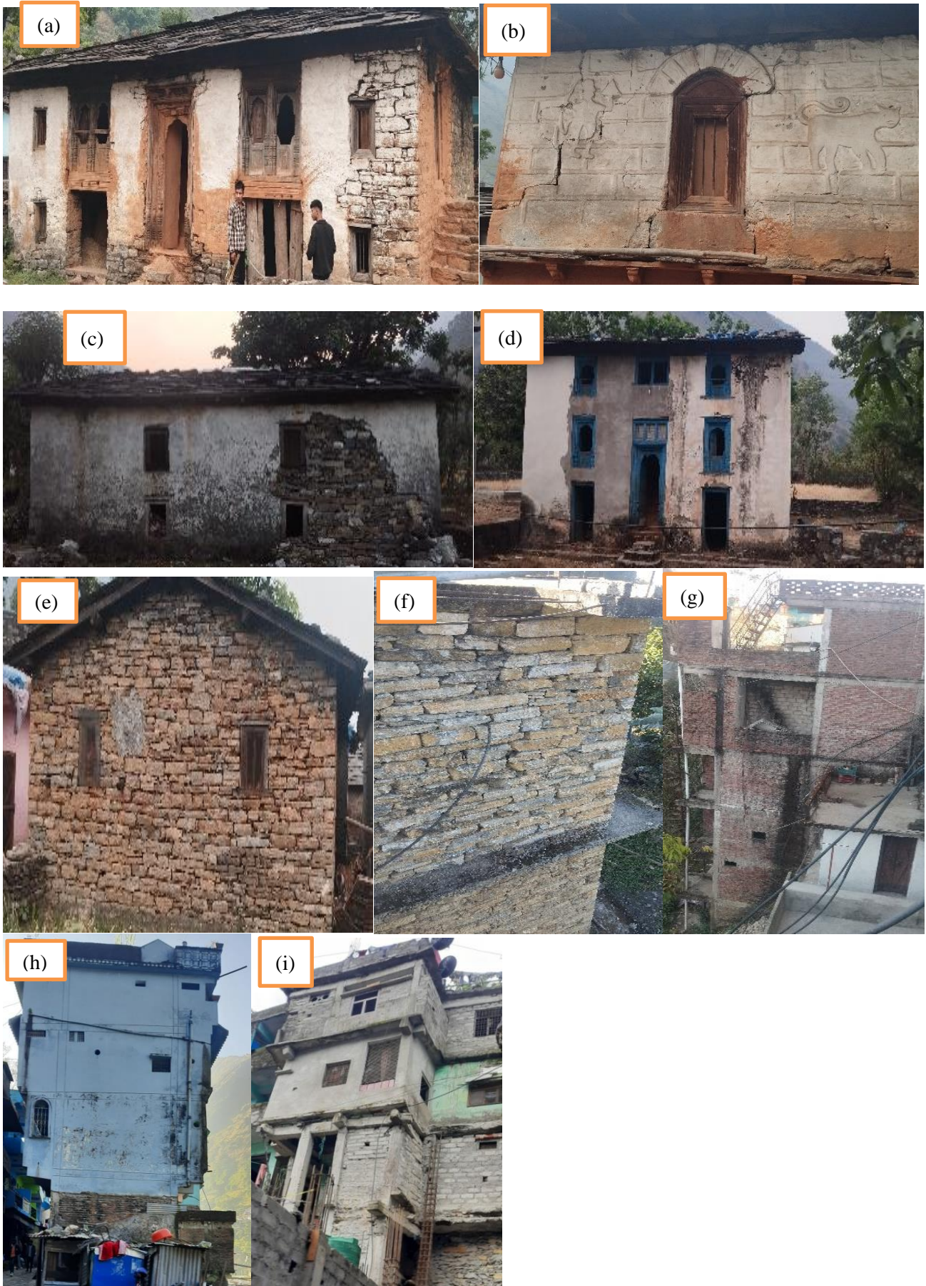
Figure 2: Common construction practice in structures in Darchula
